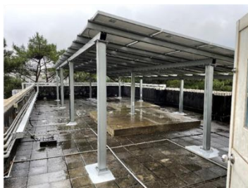
Installation of Solar Panel
